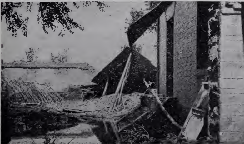
The Men's Hospital badly damaged
